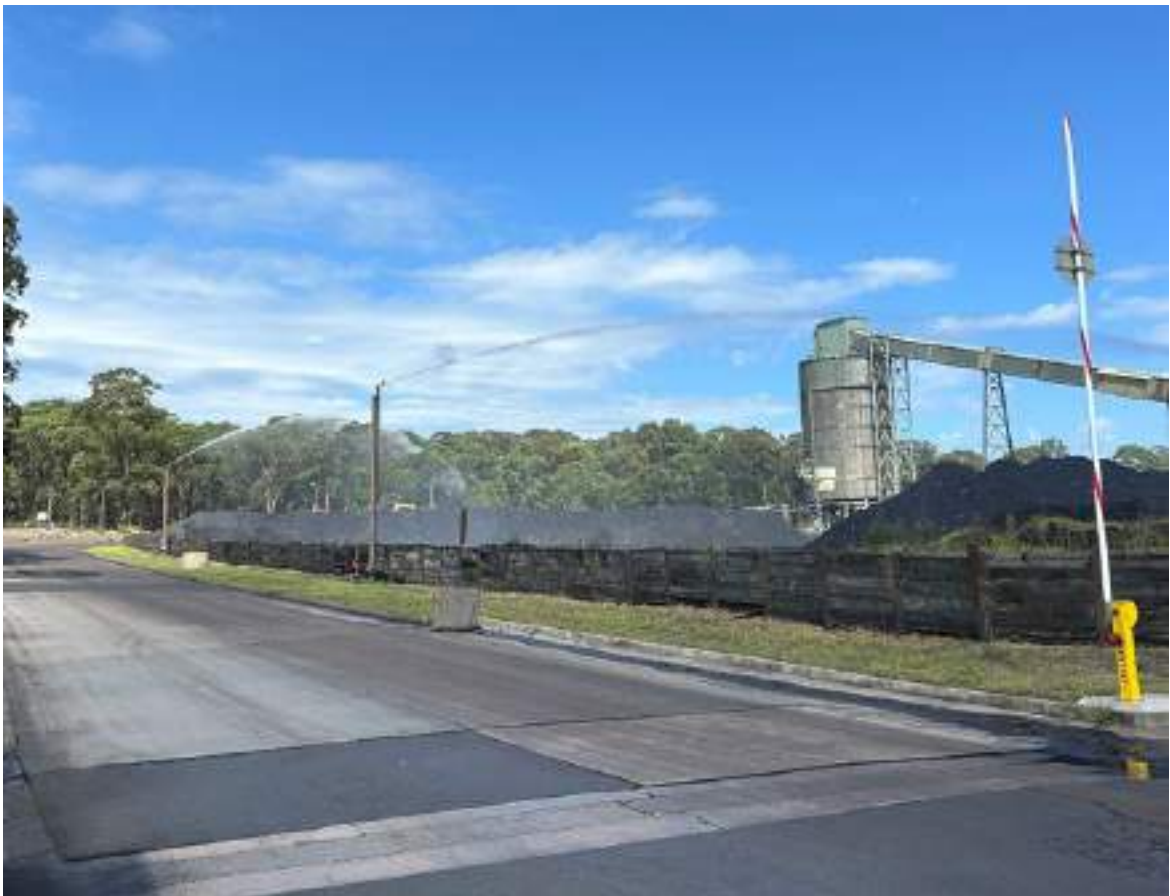
Plate 1: Appin East Stockpile Dust Suppression Sprays
