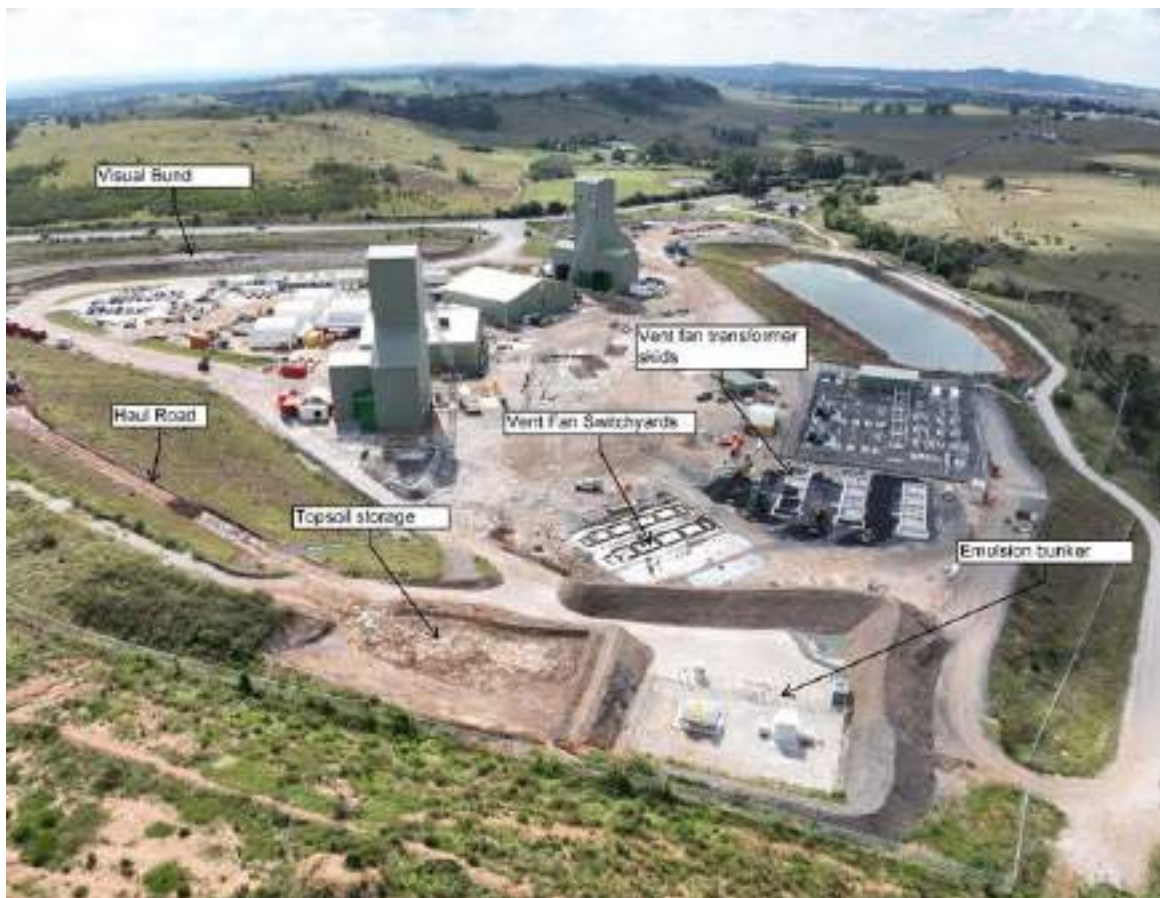
Plate 2: Aerial view of AMVA Project site under construction (April 2025)
