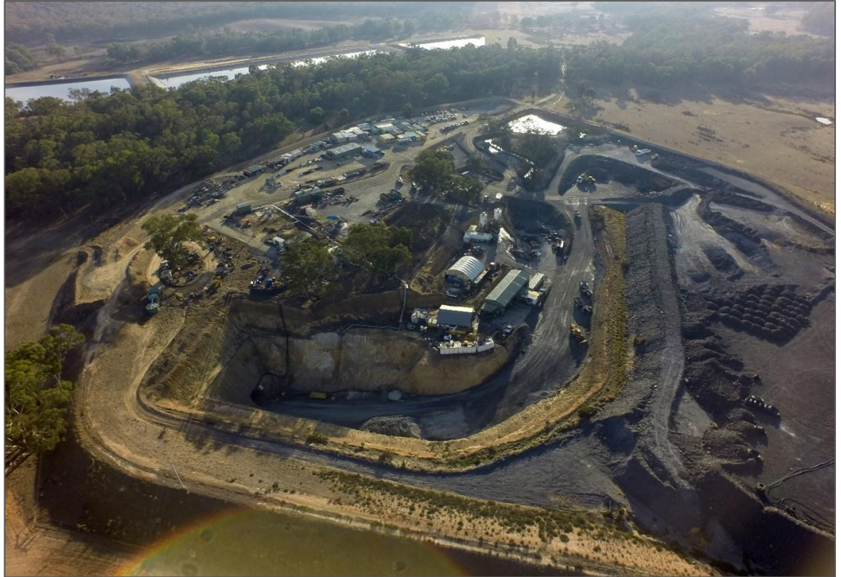
Figure 5.1: Augusta Mine site with box cut, Augusta Portal (foreground), workshop, offices and holding dams
