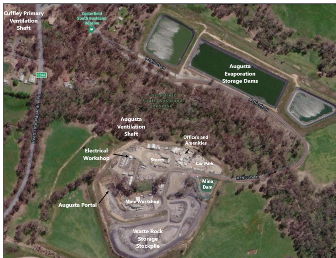
Figure 18.1: Augusta Mine site – aerial view
