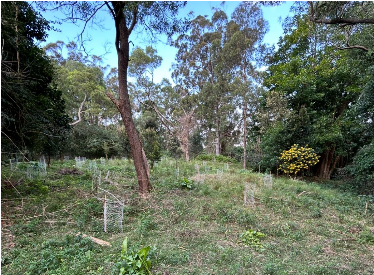
Plate 5: Dendrobium tunnel subsidence site following weed removal and tree planting
