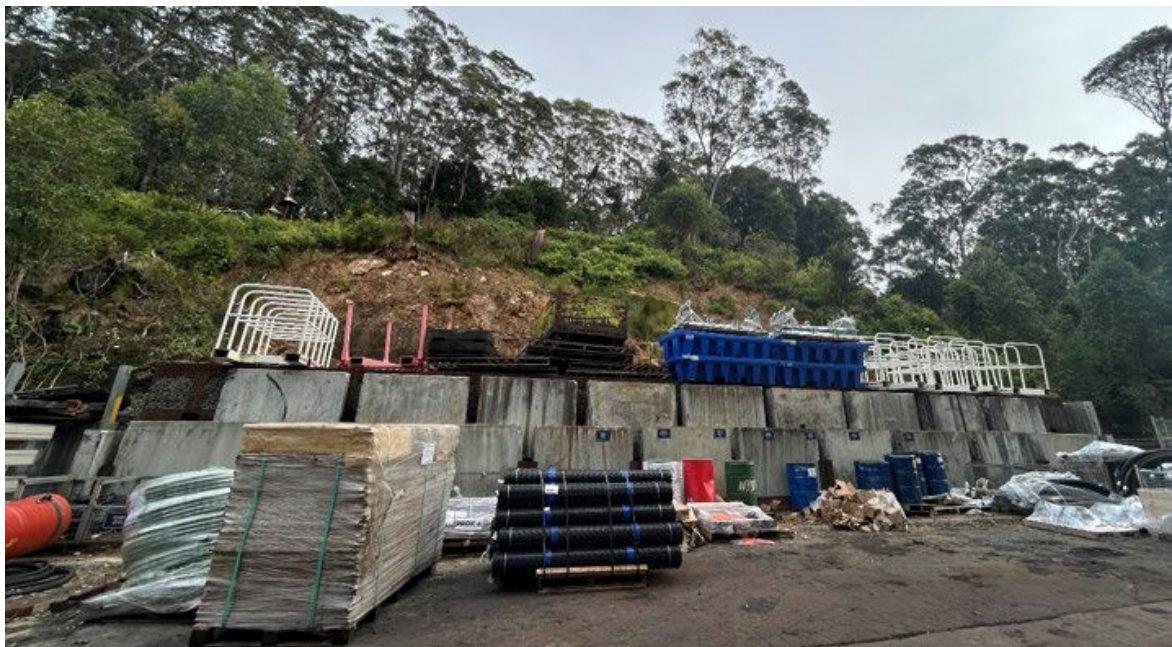
Plate 1: Slope Remediation Works – Dendrobium Pit Top Portal Road
