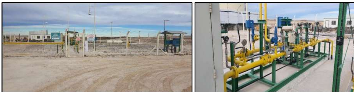
Figure 18.15: EMED plant reduces gas pressure from the General pipe line to supply generators and processing equipment on-site.
