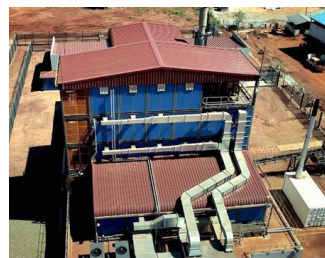
Figure M19: State-of-the-art recovery house uses UV- light to recover rubies.
