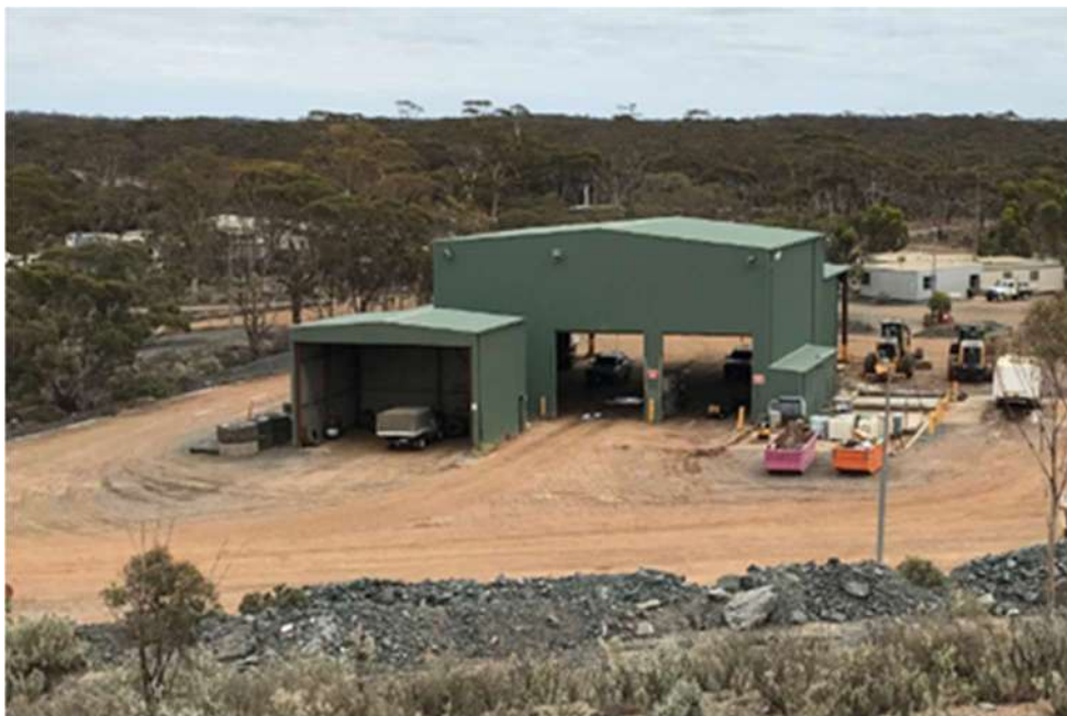
Figure 18-2 HGO Underground Workshop – Source: Westgold.
