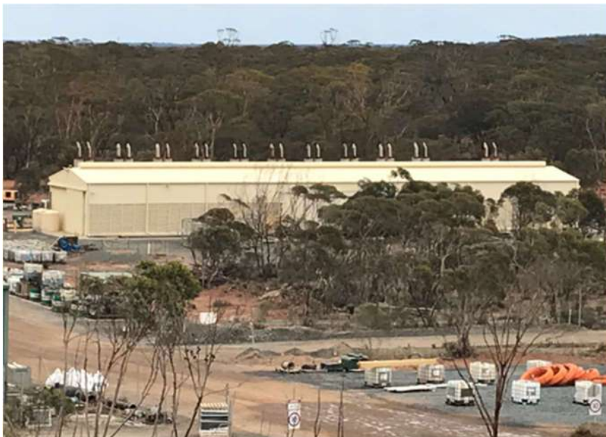
Figure 18-1 HGO Powerhouse – Source: Westgold.
