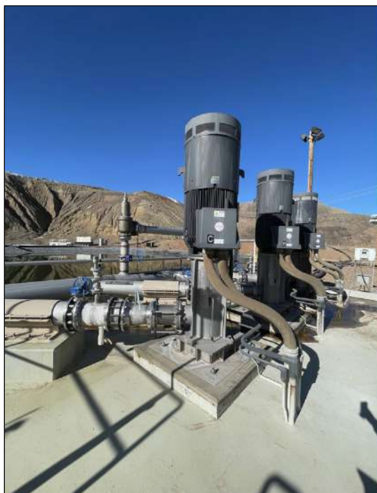
Figure 17-7: Raffinate Pumps at JCM
