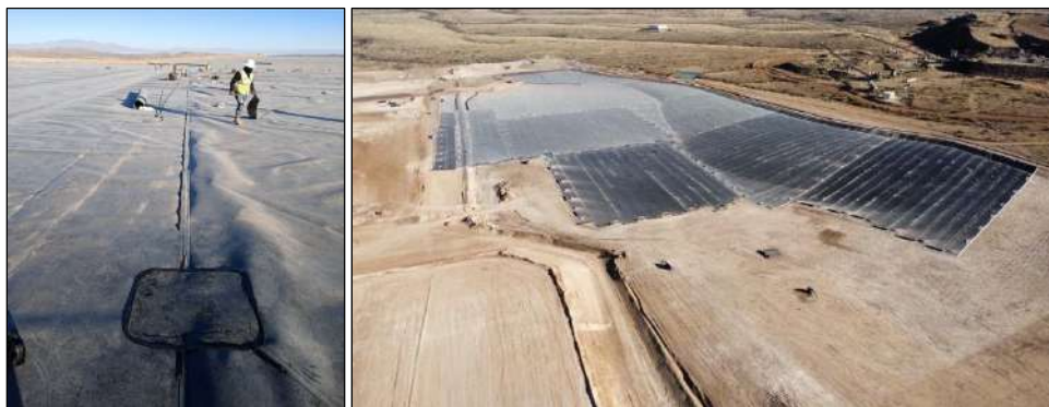
Figure 17-4: Liner Installation on Pad 5
