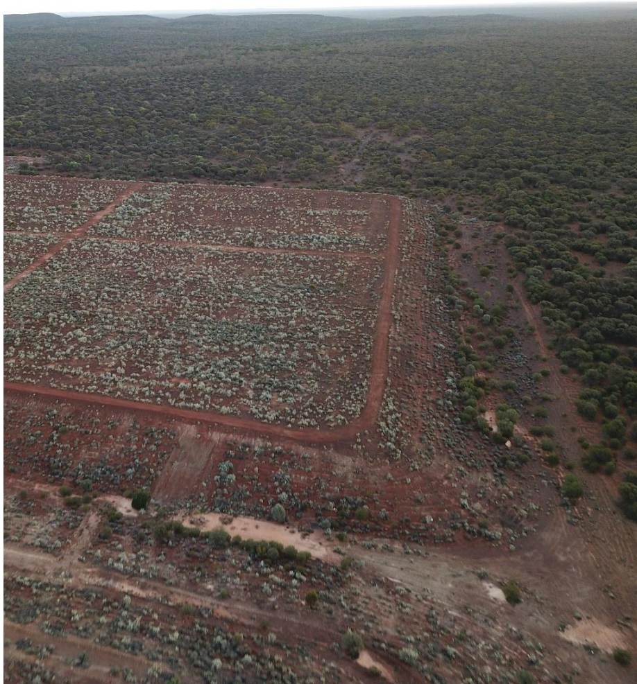
Figure 18: NorGold TSF showing ~14-degree slopes and no erosion after ~30 years
