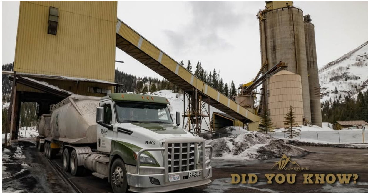
Figure C-6 – Example of the tipple at a coal mine
